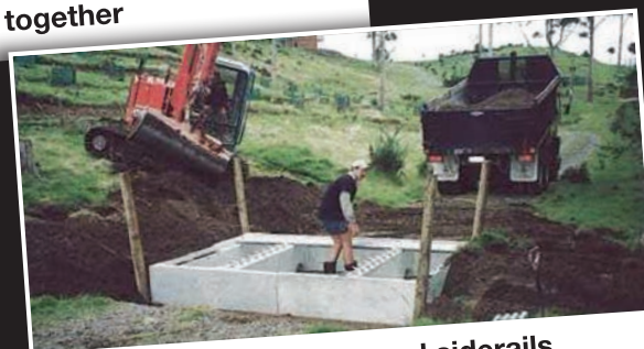
4. Backfill, place pipes and siderails
